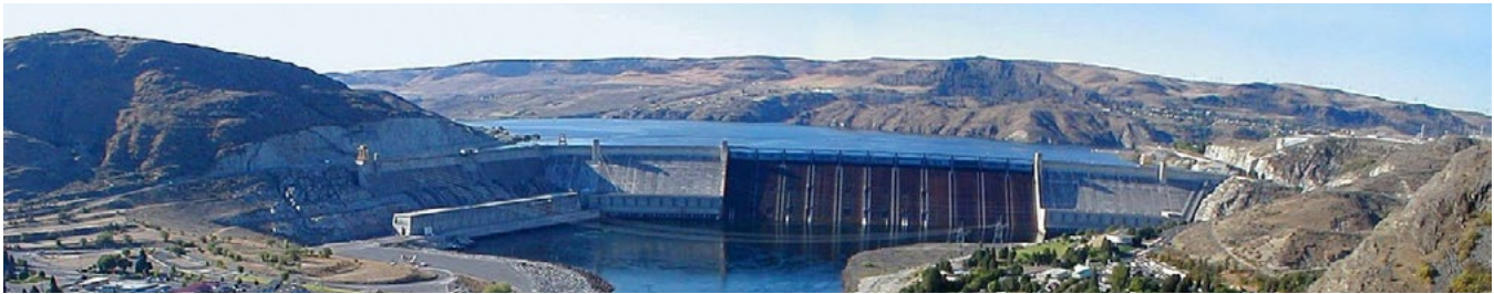
Figure 1. The GC Dam is the largest power plant on the continent.
